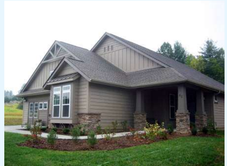
Second WaterSense labeled home built in the pilot program
