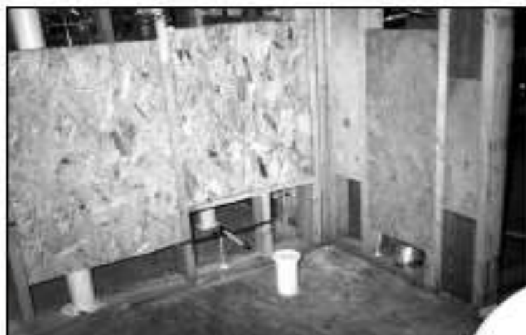
Whole wall reinforcing installed in a Habitat house
