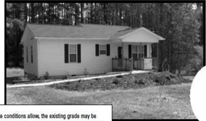
Example of a Habitat house with a gently sloping walk on an earth berm and bridge to provide a stepless entrance.
