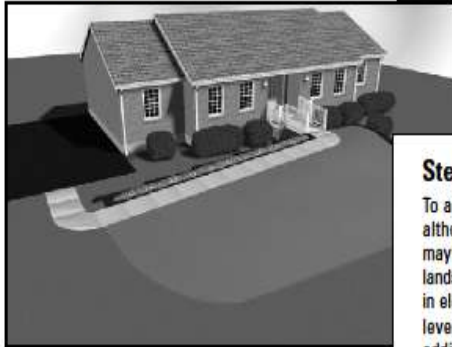
Earth berm and bridge used to achieve stepless entrance
