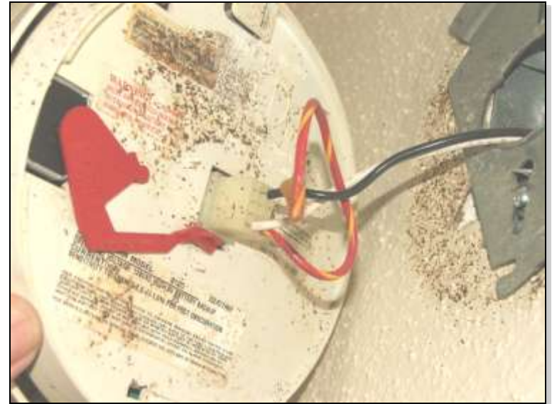
Cockroach infestation in a smoke detector
