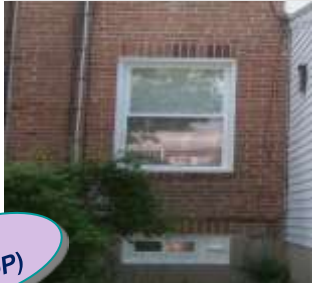
Energy Star windows installed
