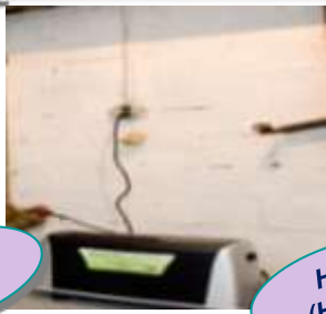
Mold remediated; dehumidifier installed
